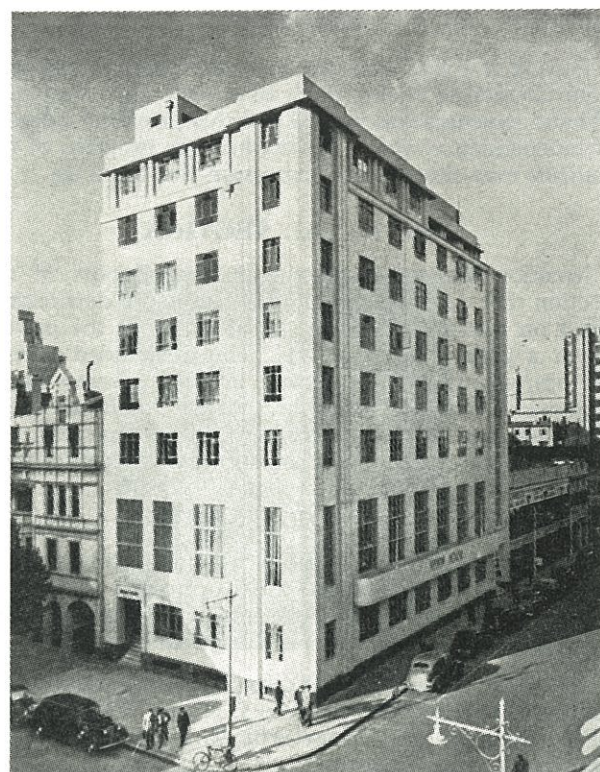
Kelvin House, Marshall Street, Johannesburg
